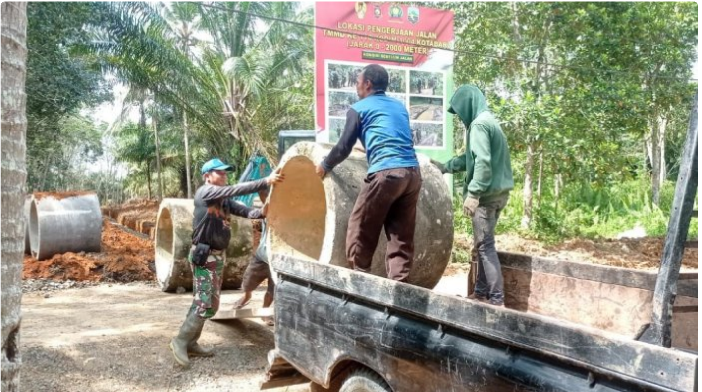
Cegah Genangan Air, Satgas TMMD ke 116 Kodim 1004 Kotabaru Pasang Gorong - Gorong
